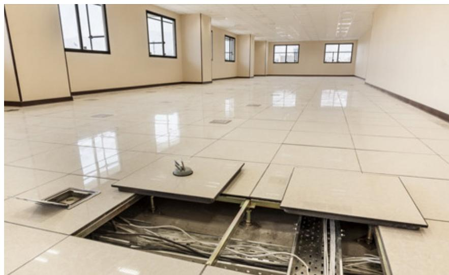
Specially designed for 600mm panel systems.
