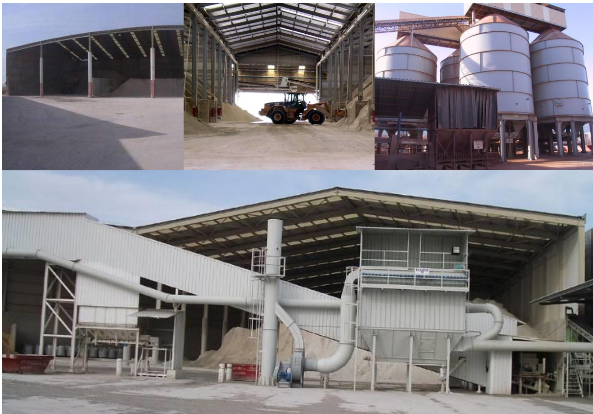
Figure 10. Examples of enclosed or semi-enclosed facilities to store dusty materials.
