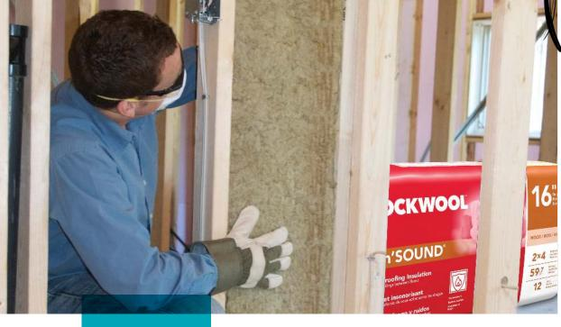
ROCKWOOL SAFE'n'SOUND® is a stone wool insulation for use in interior partitions of residential wood and steel stud construction where superior fire resistance and acoustical performance are required.
